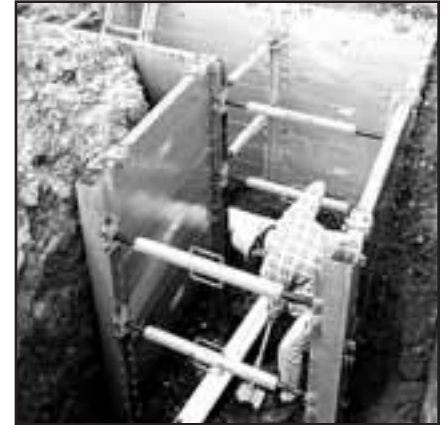
Two-Sided corner configuration with adjustable spreader struts and full length corner posts
