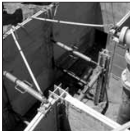
Three-Way "T" Configuration with adjustable spreader struts and combination t-posts and 4-way posts
