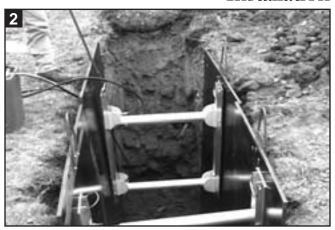
Release the top rail and allow shore to completely unfold. The shore will lock itself into open position.
