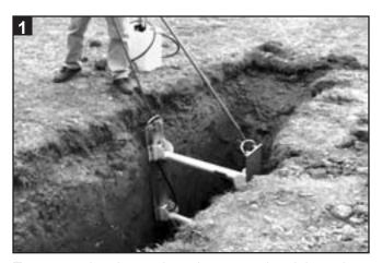
To remove the shore, place the removal tool through the handle with the hook facing the trench. Place the end of the tool over the same fitting where hose was hooked.
